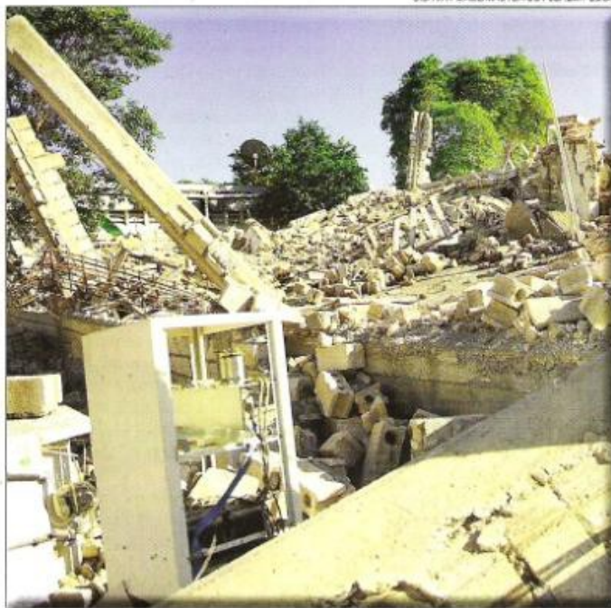
Shown here are destroyed buildings in Jacmel, Haiti. According to local officials about 350 people lost their lives in Jacmel due to the earthquake that hit the region January 12, 2010.
